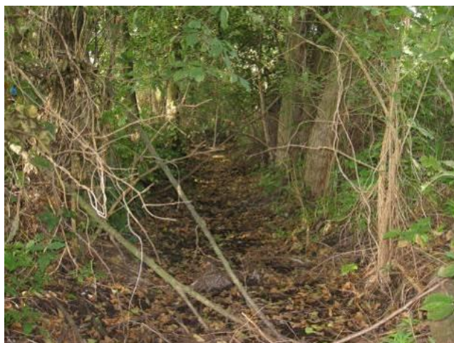
Figure 1 Clogged regulated riverbed of Porec overgrown with vegetation
