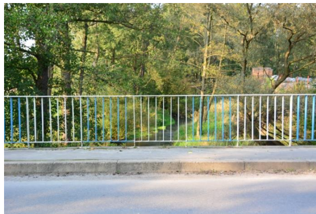
Figure 4. Engineering constructions on the river Dłubnia (Bridge in Michałowice).
