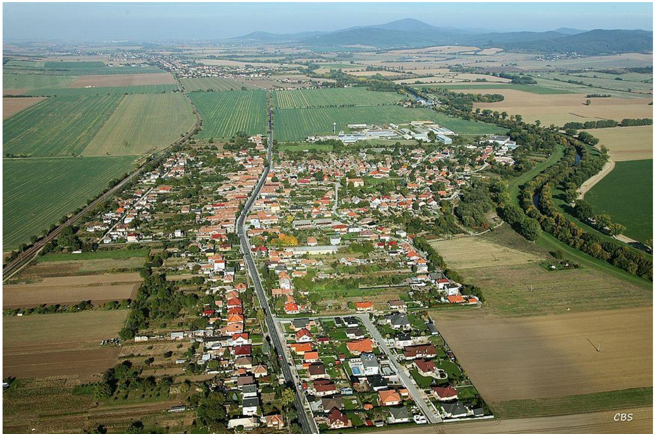
Figure 1 Jelšovce (source: http://www.jelsovce.sk/typo3temp/pics/85a3054ffe.jpg )
