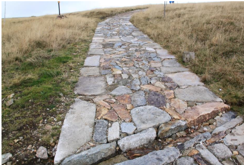
Figure 6 layout of the stone base trail – border field filled with vertically wedged stones (source: author)
