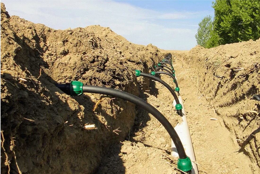
Picture 61 Underground irrigation piping (irrigators.org.au)
