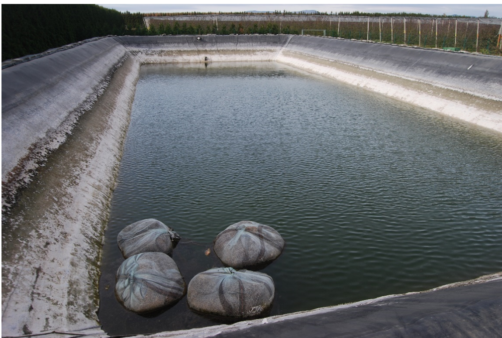
Picture 60 A pool with rain water collected from the roofs of adjacent storage halls serves for drip irrigation in the orchard nearby in Plantex, Veselé pri Piešťanoch Ltd., SK (Paulen)
