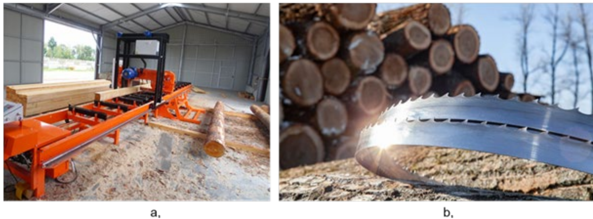
Figure 1 Work in the sawmill on a log saw (a.); saw bands (b.)
